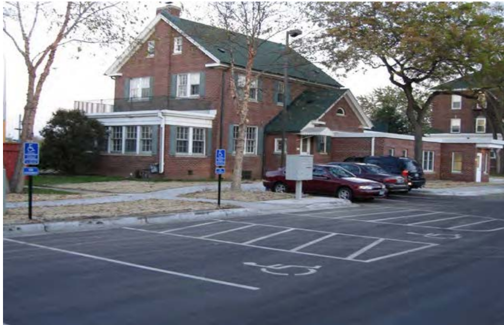
VICTRI in Building 11 at the Minneapolis VA Medical Center Campus
